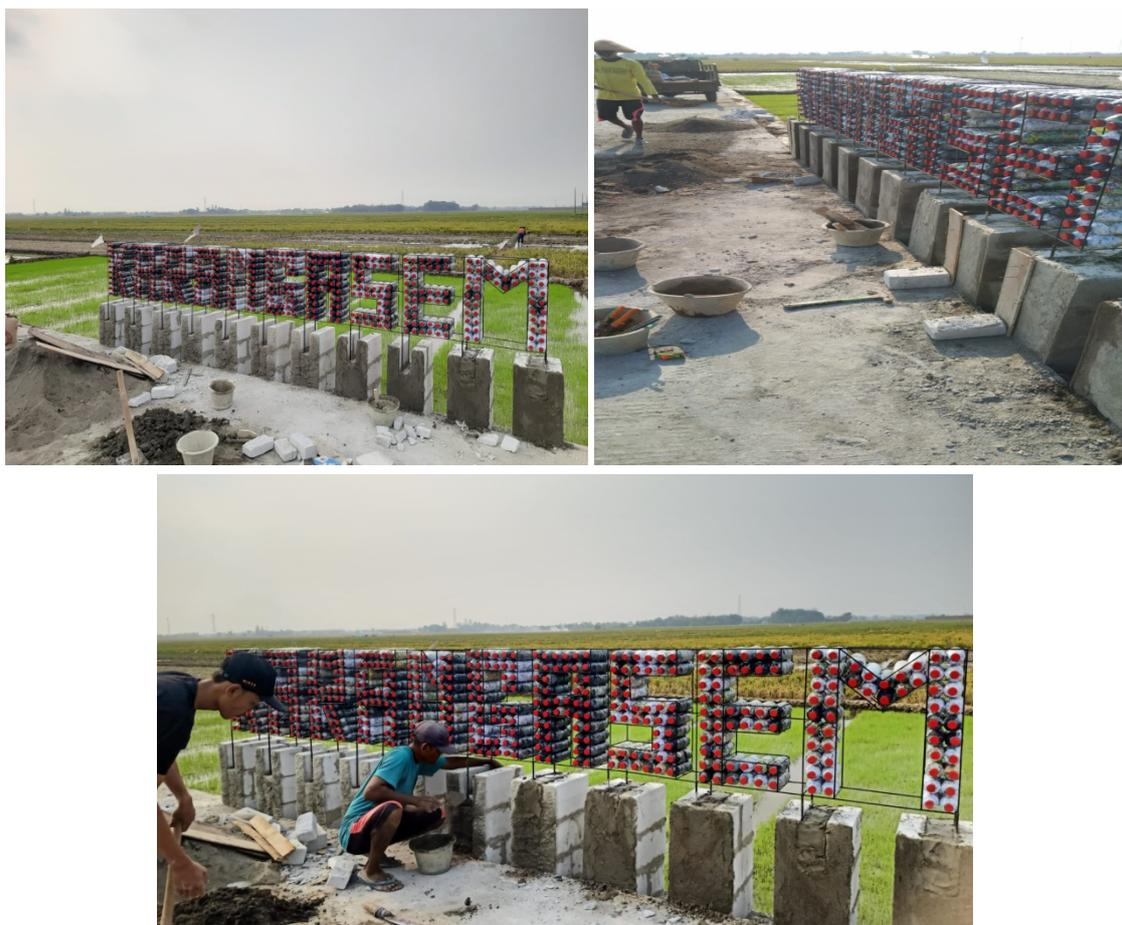
**Gambar 10.** Pemasangan pondasi landmark ecobrick
